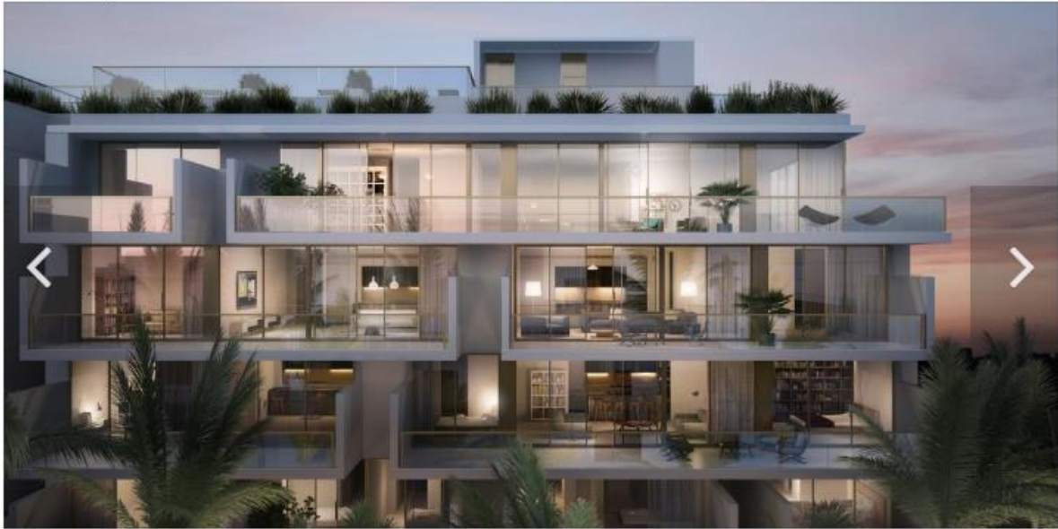
JMH Development's 300 Collins in Miami Beach has 19 condos under construction.
